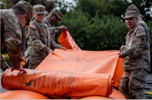
Florida Army National Guard soldiers help deploy a flood mitigation device to protect a hospital from flooding in Sanford, Fla., on Oct. 8. (Photo by Sgt. Marc Morgenstern/Army)
